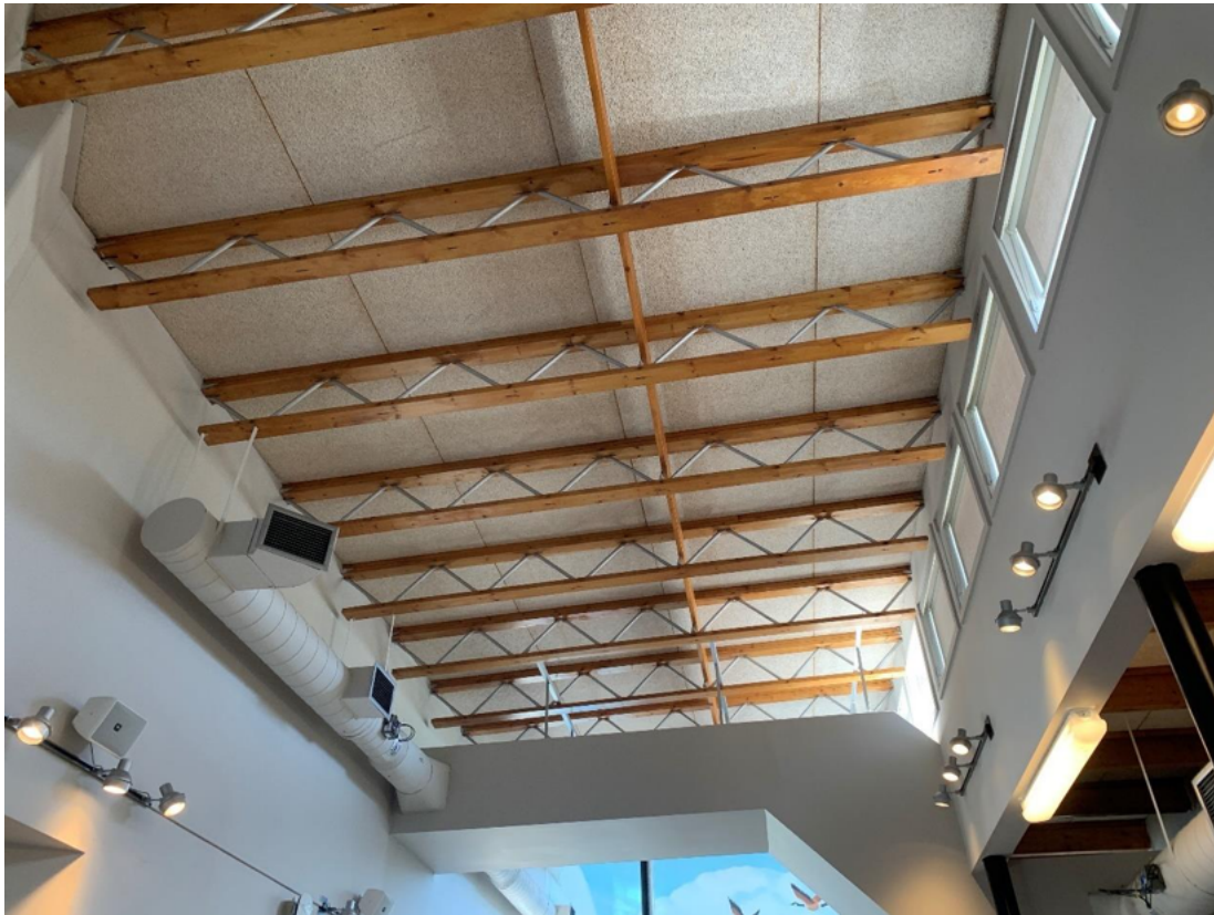
Figure 4: Roof Area B structure
