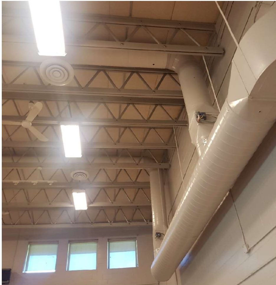
Figure 13 Auditorium VAV system
