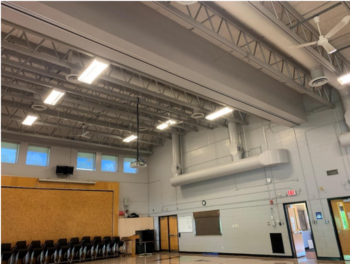
Figure 3: Roof area A parallel chord trusses.
