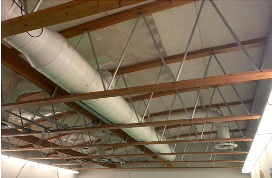
Figure 5: Roof Area E structure.
